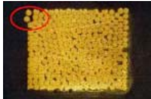
Figure 4.3.5.a Example cross sectional view of an un-acceptable weld due to strands not in contact with the weld bond.
